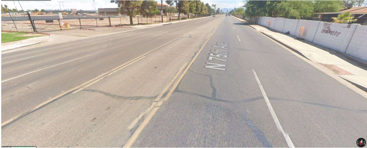
Figure 1: Existing ADA compliant curb ramps are provided along both directions of N 75 th Avenue.
